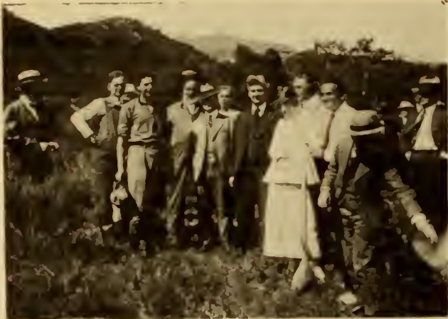
Lillian Gish and Mayor Sebastian Breaking Ground for Stadium.
